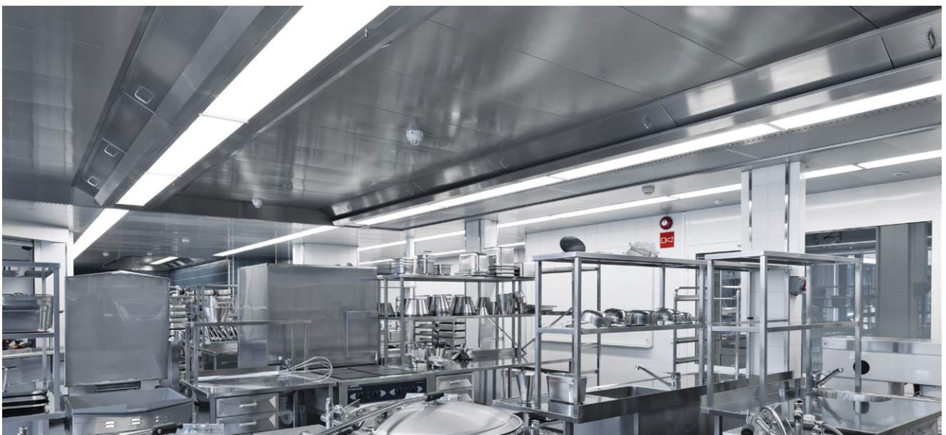
Kotka central kitchen (Kotka, Finland)
