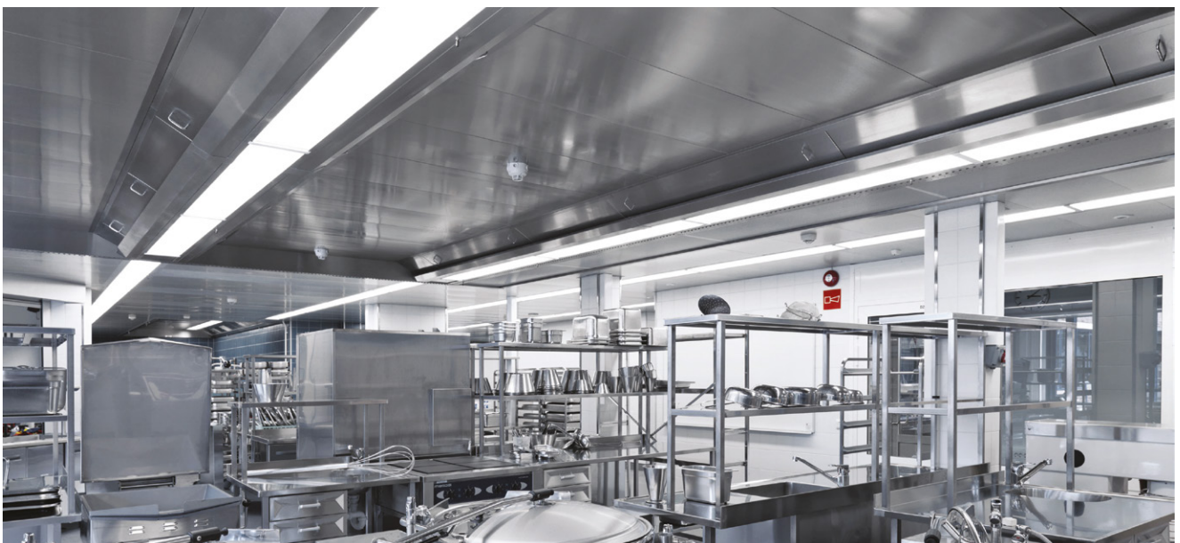
Kotka central kitchen (Kotka, Finland)
