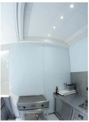
Project: Product: Zeppelin Baumaschinen, Garching, Germany KCW (Clean) vaulted ventilated ceiling, Jet Extraction system (JES), low velocity design supply unit
