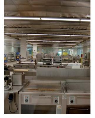
Project: Bangkok Air Catering, Bangkok Product: KCJ (Inter) ventilated ceiling Special feature: Special large surface ceiling Exhaust airflow rate: 169,000 m³/h Surface area: 1,360 m²
