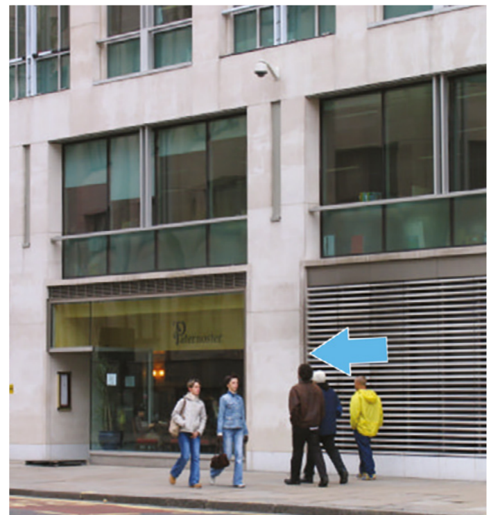
Dion and Pater Noster restaurants (London) whose kitchens are equipped with one PolluStop PEU unit. Discharge points are on the building fronts.
